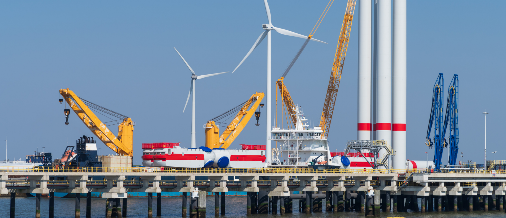
Offshore vessel for placing wind turbines at sea in the Eemshaven harbor. Groningen, Holland.
